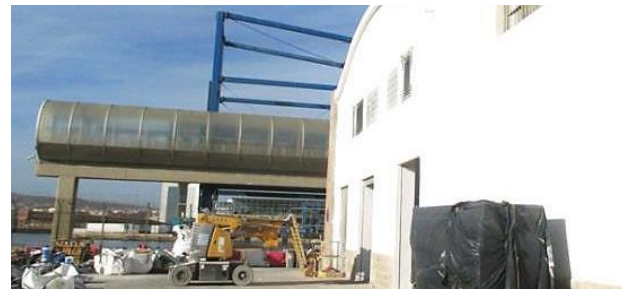
New building of the shed n°5
