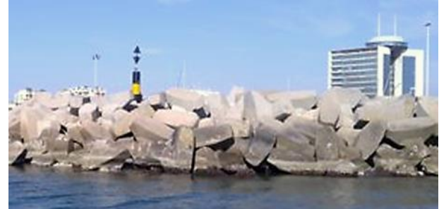
Supply and installation of basis for beacons
