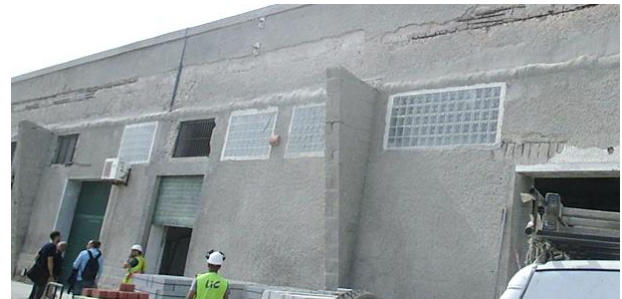
Renovation and repair of the perimetral hoop
